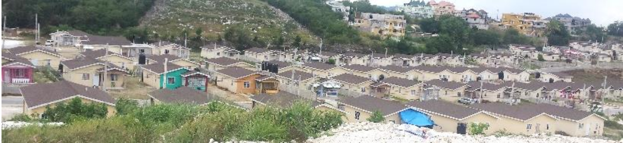
Phase 2 : 300, 1 & 2 Bedroom homes(Under Construction)
